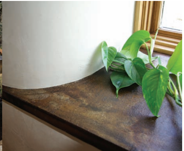
Exterior clay render with earthen pigment (left). Interior clay plaster and custom concrete countertop accent the deep window sill of this strawbale wall (right).
